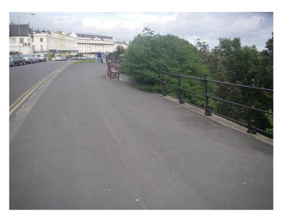
Plate 75 Scarborough South Cliff. Promenade showing signs of subsidence.
