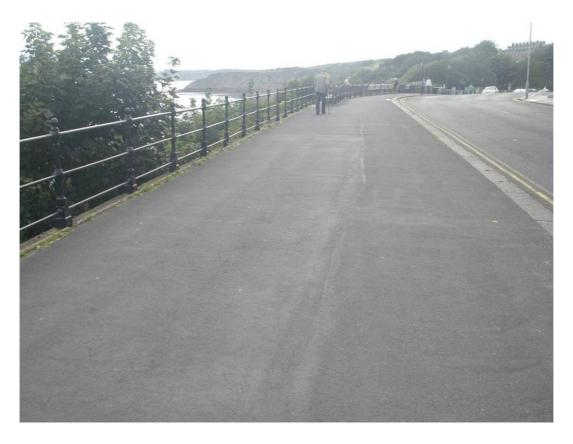
Plate 76 Scarborough South Cliff. Promenade showing signs of subsidence.
