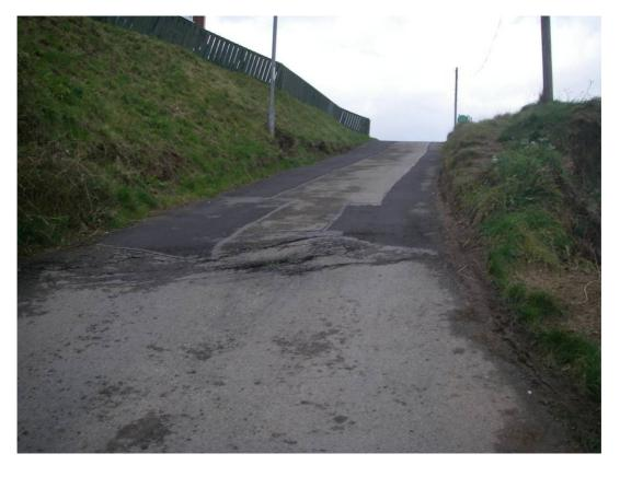
Plate 29 Site view of tension cracks and bulge in access road into Flat Cliffs.
