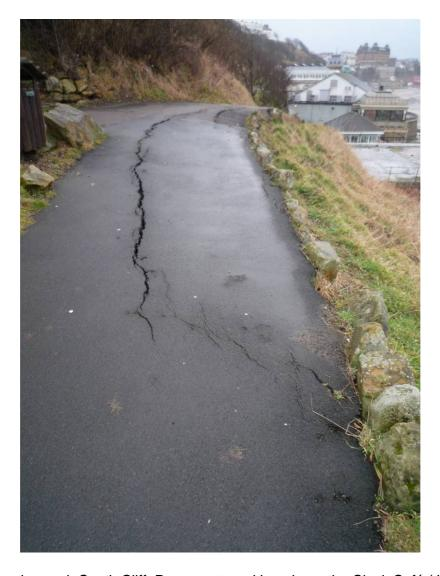
Plate 80 Scarborough South Cliff. Pavement cracking above the Clock Café (Jan. 2010).
