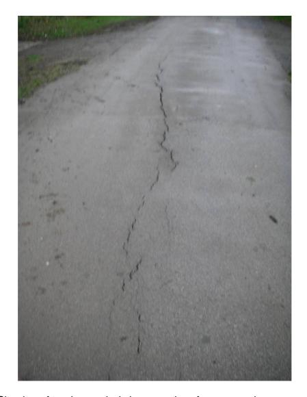
Plate 32 Site view of tension cracks in lower section of access road (Dated 27<sup>th</sup> Nov 2008)
