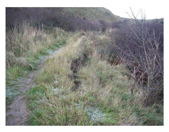
Plate 9 Site view of mid-slope back rotated block and surface tension cracking (November 2008).
