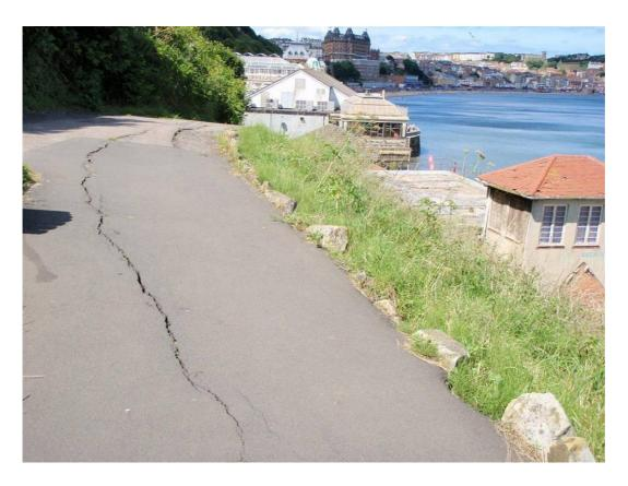
Plate 77 Scarborough South Cliff. Pavement cracking above the Clock Café (July 2008).
