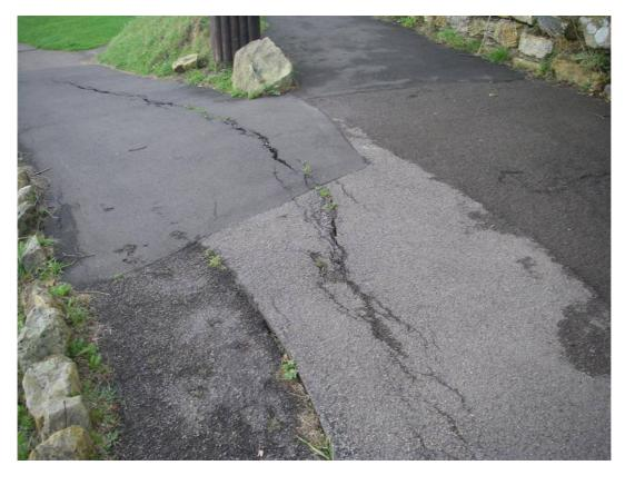
Plate 78 Scarborough South Cliff. Pavement cracking above the Clock Café (Sept 2008)
