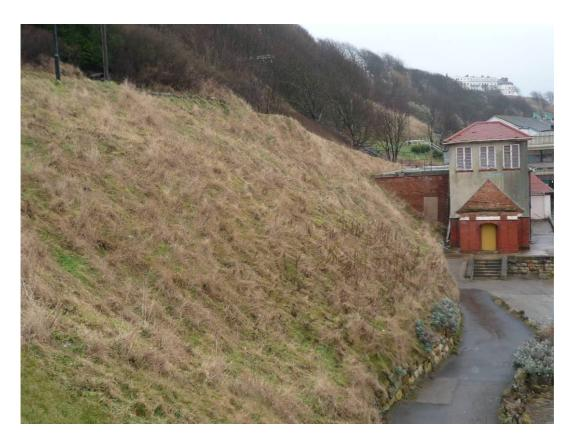
Plate 81 Scarborough South Cliff Slope bulging adjacent the Clock Café (Jan 2010).
