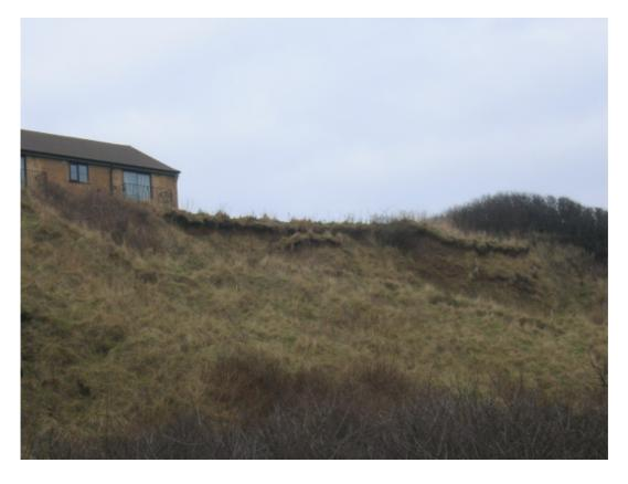
Plate 8 Site view of Behaviour Unit II showing increased degradation and collapse of over-steepened back-scarp below Upper Plateau (January 2010).
