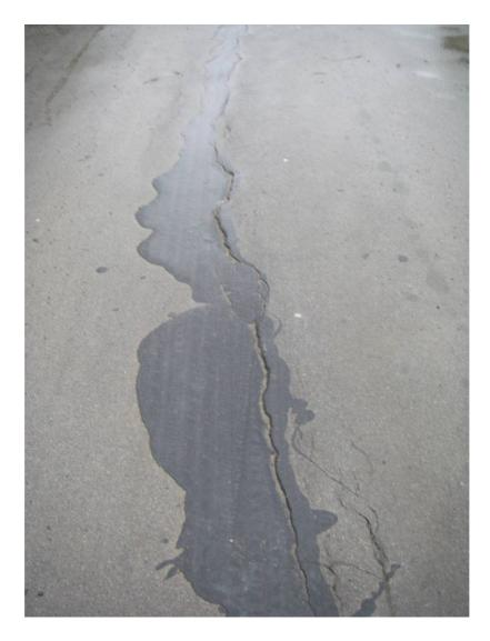
Plate 33 Site view of repair to tension cracks in lower section of access road (Dated 12<sup>th</sup> Jan 2010).
