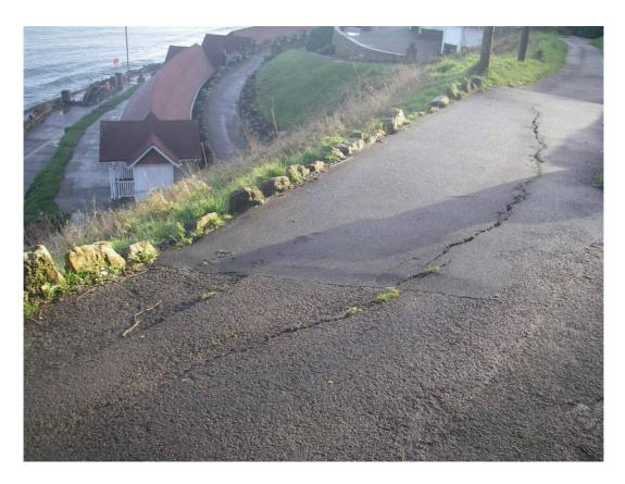
Plate 79 Scarborough South Cliff. Pavement cracking above the Clock Café (Dec 2008)
