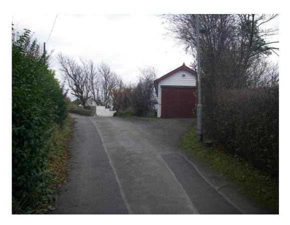
Plate 30 Site view of leaning timber garage at No. 5 Flat Cliffs; seaward of coastal slopes.
